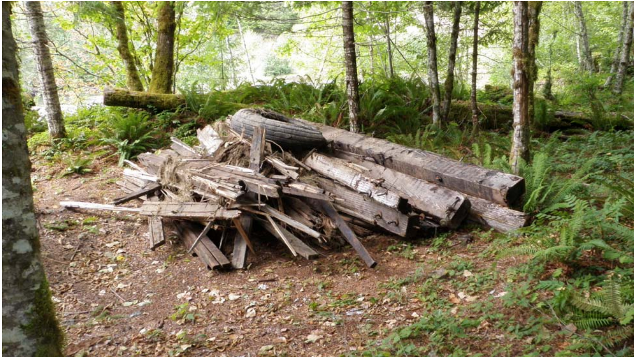
Figure 1. Picture of some of the creosote timbers removed from the logjam. Timbers were disposed of properly at a hazardous waste facility
