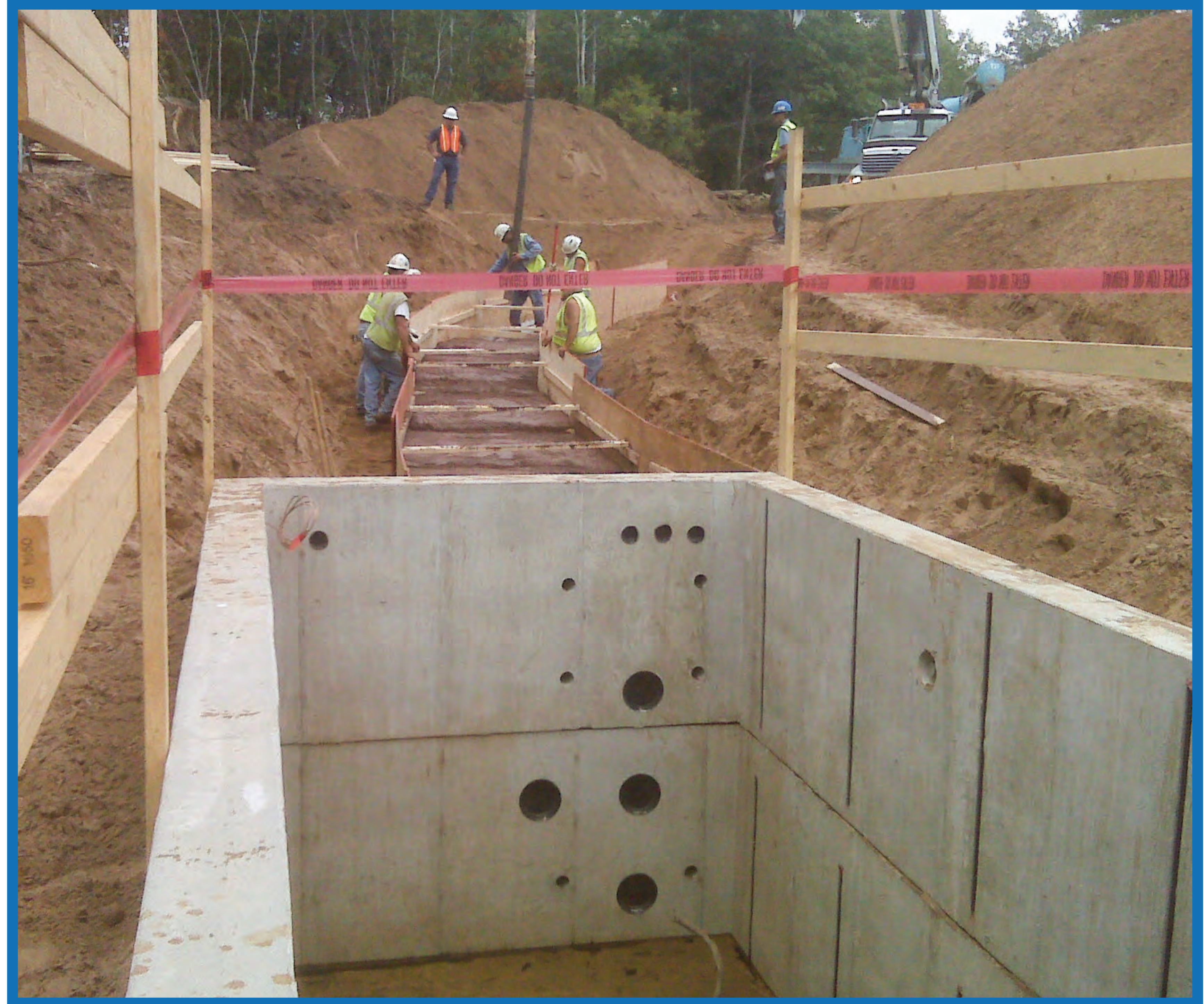
Concrete access vault for transmission line
