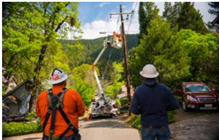
Figure 46: Lineworkers Performing Work
