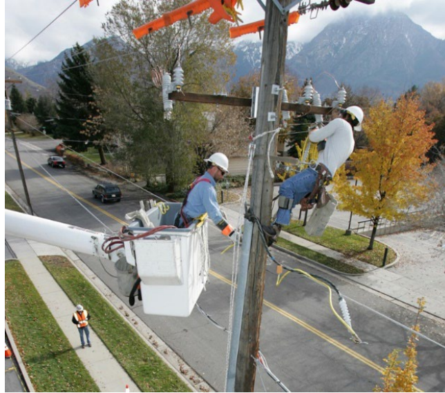
Figure 29: Lineworkers Preparing a Pole for New Covered Conductor
