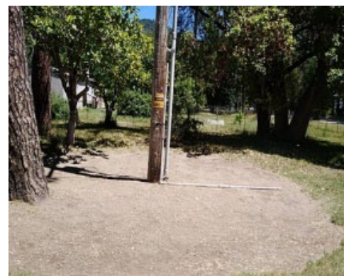
Figure 36: Pole Clearing at Pole Base
