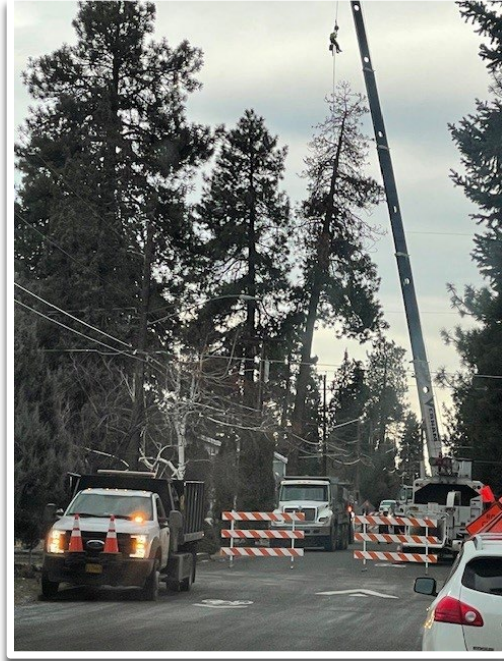
Figure 15: High-Risk Tree Removal
