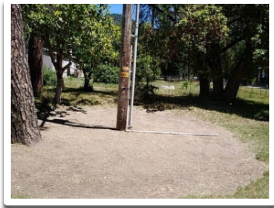
Figure 17: Pole Clearing at Pole Base
