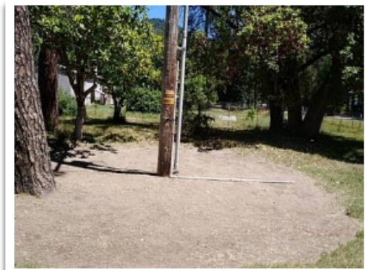
Figure 17: Pole Clearing at Pole Base
