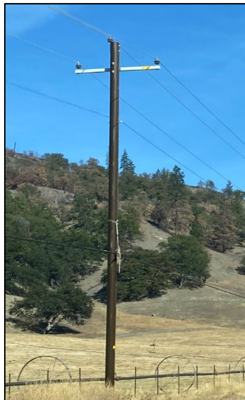
Figure 19: Distribution Fiberglass Poles
