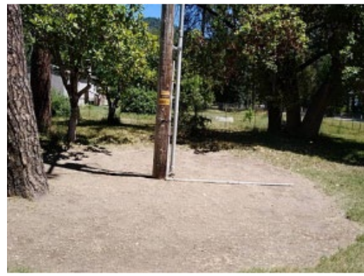
Figure 20: Pole Clearing at Pole Base
