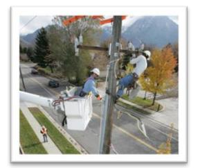
Figure 18: Lineworkers Preparing a Pole for New Covered Conductor
