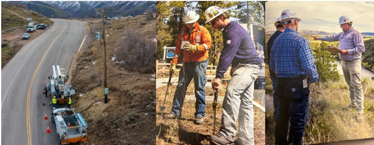
Figure 6-1: Line Workers Performing Field Work
