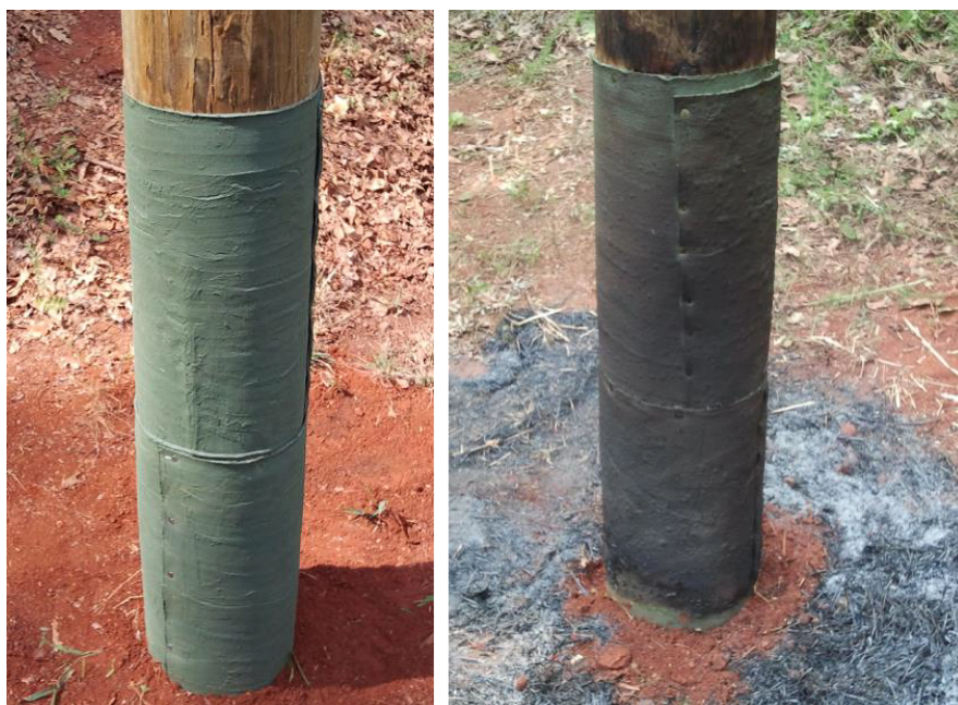
Figure 2—Example of Finished Application
