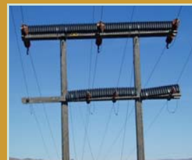
Nest discouragers (PVC pipe and drain pipe)
