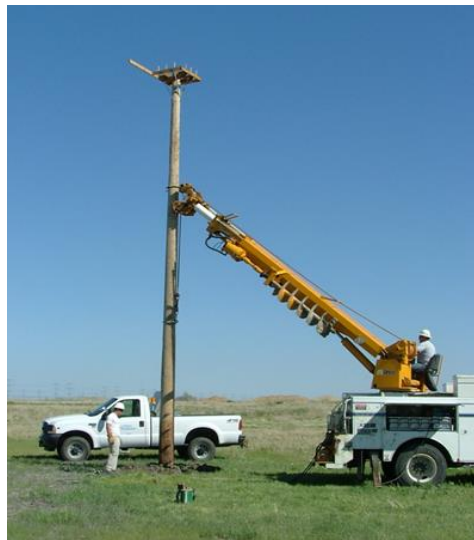
Separate pole with nest platform
