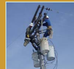
Retrofitting nearby pole
